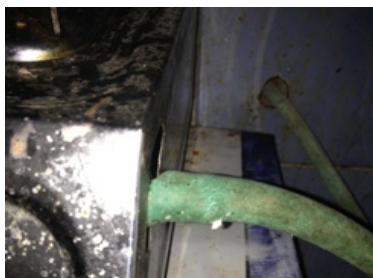
Picture 1 Rubber hose connected to biogas stove
