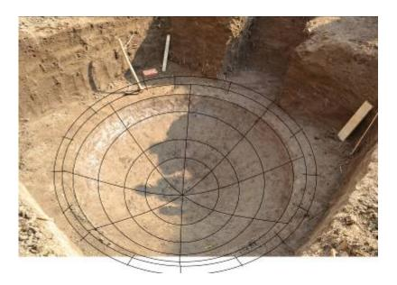
Concrete is poured into the curved pit and over the shoulder and smoothed to an even depth of 30 mm. The steel work is placed on the concrete and another 40 mm poured over it. The concrete needs to be well compacted to remove voids before it starts to set. The concrete should be cured, by keeping it wet with water for four days, before any further building work is started. This approach will prevent any problems caused by the soil shifting.
